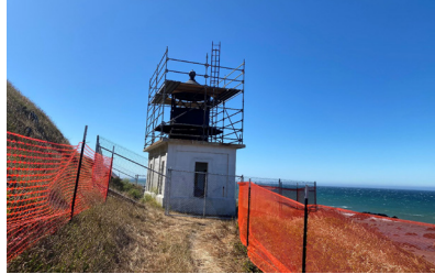
Scaffolding of the lighthouse
