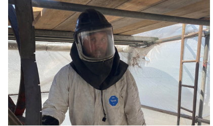
Sponge jetting activities
