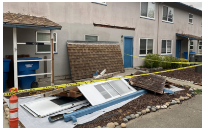
Initial demolition of non-hazardous front awnings
