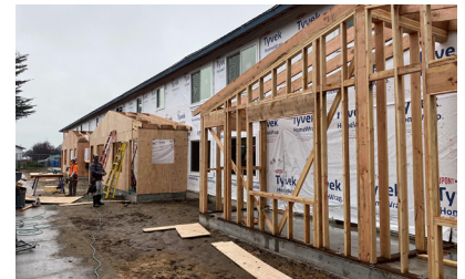
Construction of front enclosures
