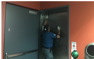
Emergency opening of elevator doors
