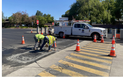
Ground loop installation
