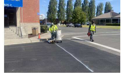
Thermoplastic restriping
