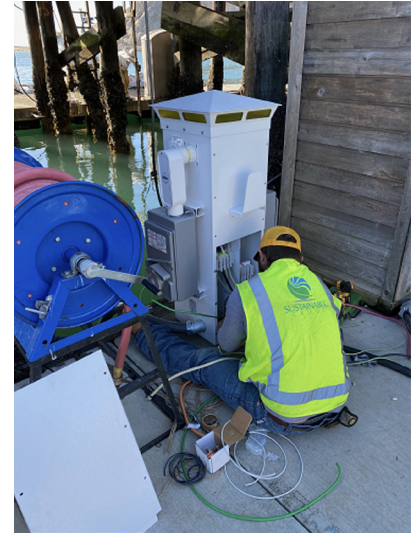
Wiring of the new electrical shore tie pedestals
