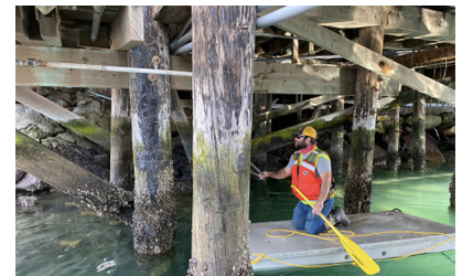
Installation of conduits under pier
