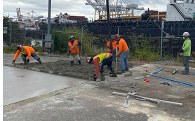
Concrete placement over sinkhole area
