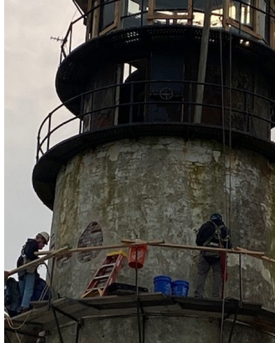
Stucco repairs
