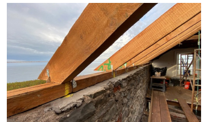
Roof framing repairs
