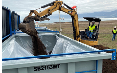
Placing of soil in lined bins
