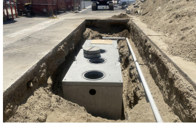
New tank and temporary by-pass line installed
